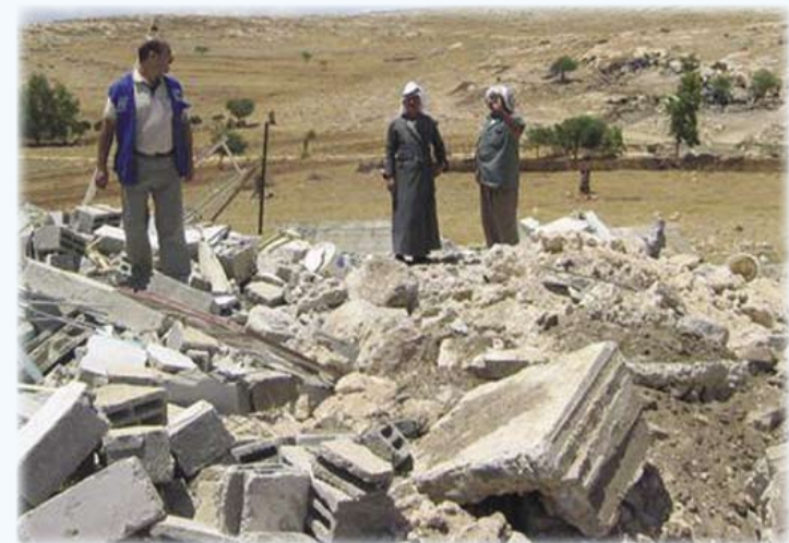
Rubble of demolished school, Khirbet Tana, Nablus.
