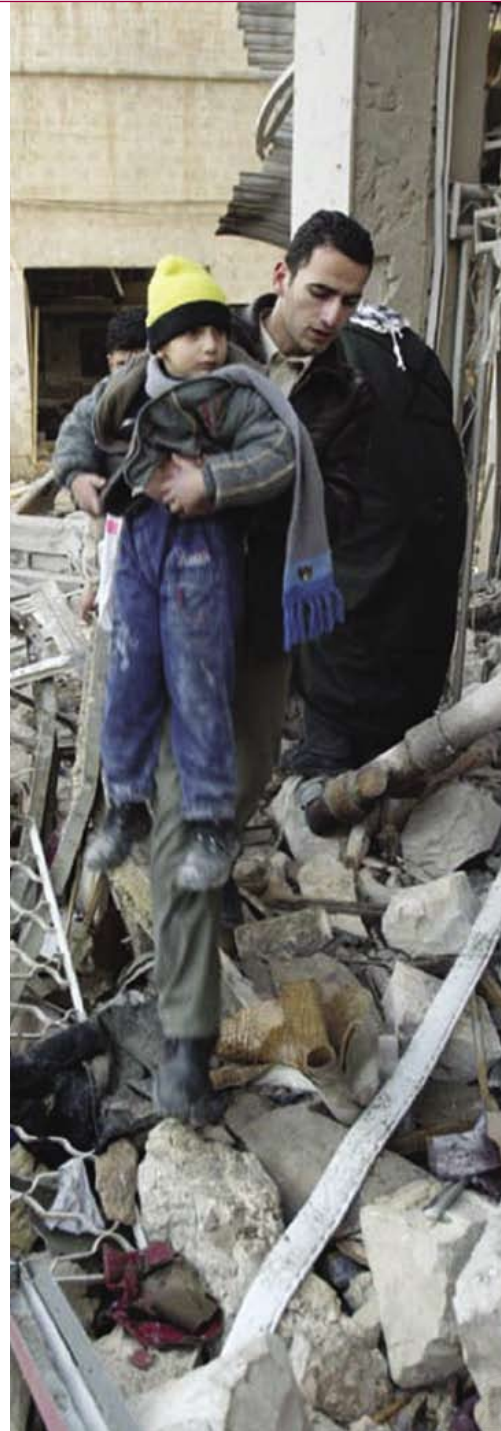
Shakaa house demolition, Nablus. Photo by Adid Qasini, March 2005
