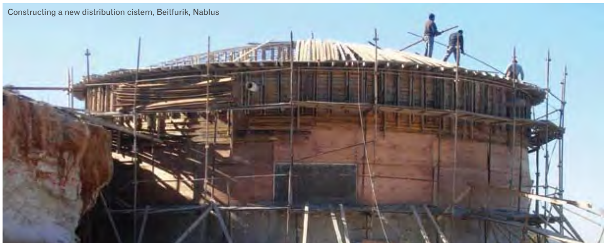
Constructing a new distribution cistern, Beitfurik, Nablus
